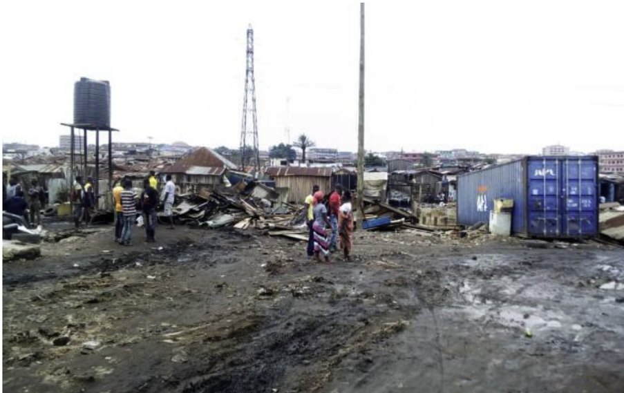
Fig. 1. Demolished (illegal) structures in waterways by city authorities in Kumasi.
